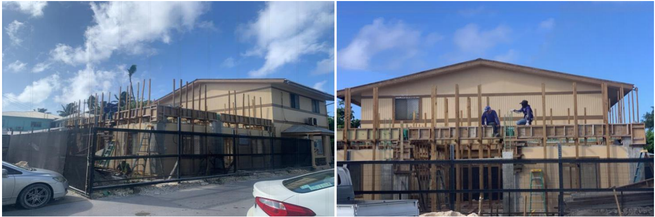
OFFICE REPAIR/EXPANSION PROJECT
