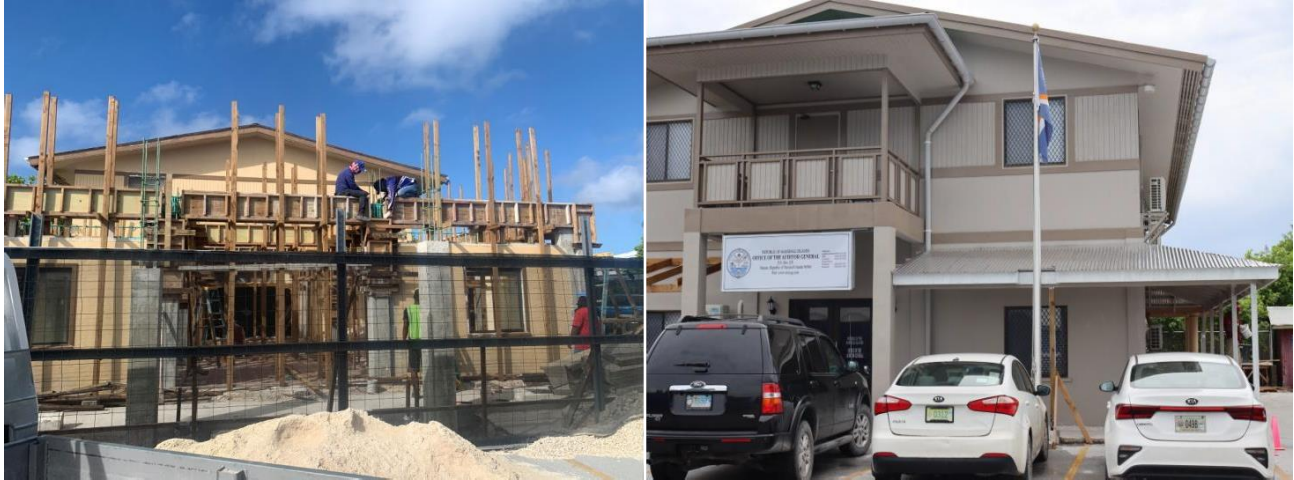
OAG REPAIR & EXTENSION PROJECT - PROGRESS PHOTOS
